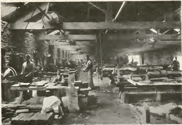
Splitting and dressing Slates, Blaenau Festiniog
